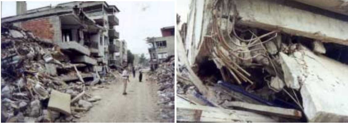
Extensive damage to buildings in Adapazari (left), poorly confined reinforcement (right)
