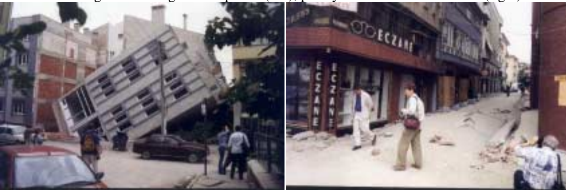
Typical liquefaction effects : overturned building (left), settlement of buildings (right)
