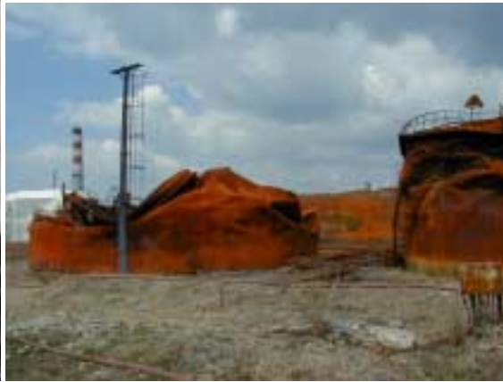
TUPRAS refinery broken chimney (left), burned and collapsed tanks (right)
