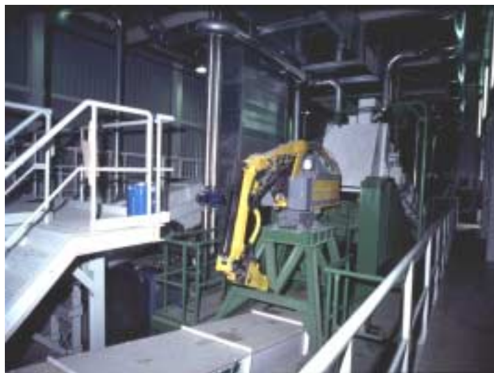
Figure 4. General view of the concrete crushing and sampling facility
