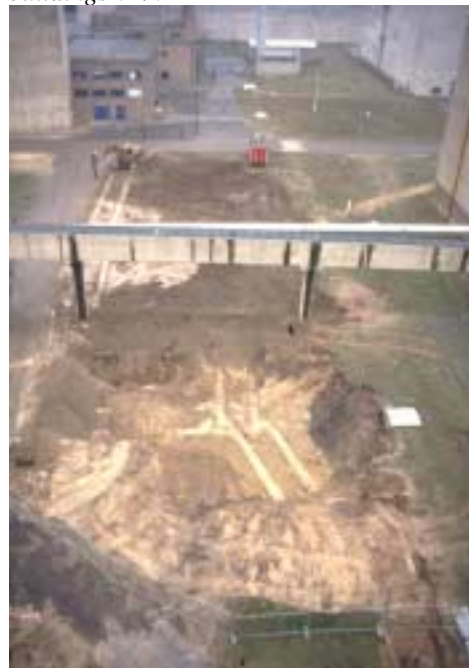
Figure 2. Green field conditions after demolition of buildings 6A/6B
