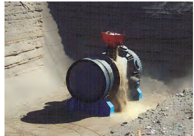
► Disposal of the reactor pressure vessel from the Trojan NPP. Richland disposal facility for radioactive waste, Washington, USA. [Photo: US Ecology, Inc.]
