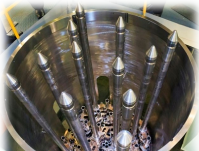
Assembling the upper core support structure
