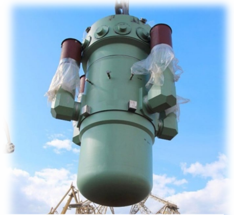
Installing the RITM-200 steam generating unit
