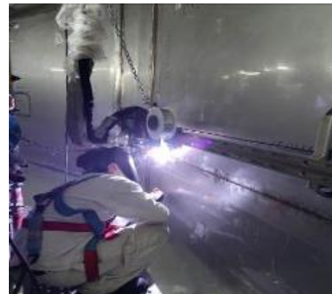
Automatic welding of SFP
