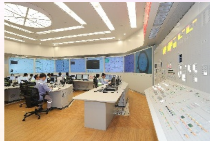
2019-4-27 Cold hydrostatic test completed for FuQing 5
