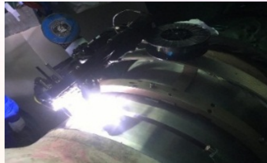
2019-6-24 Main pipeline welding completed For FuQing6
