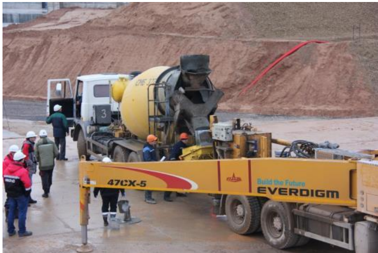
First Concrete for Unit 1 November 2013
