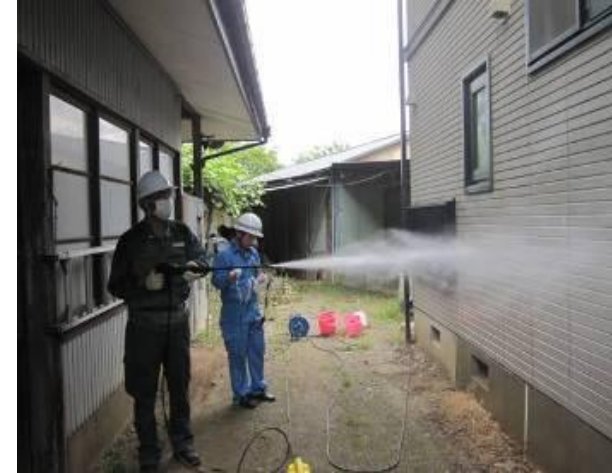
Wash wall with high-pressure water
