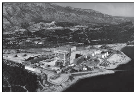
Vandellos-I before dismantling.
