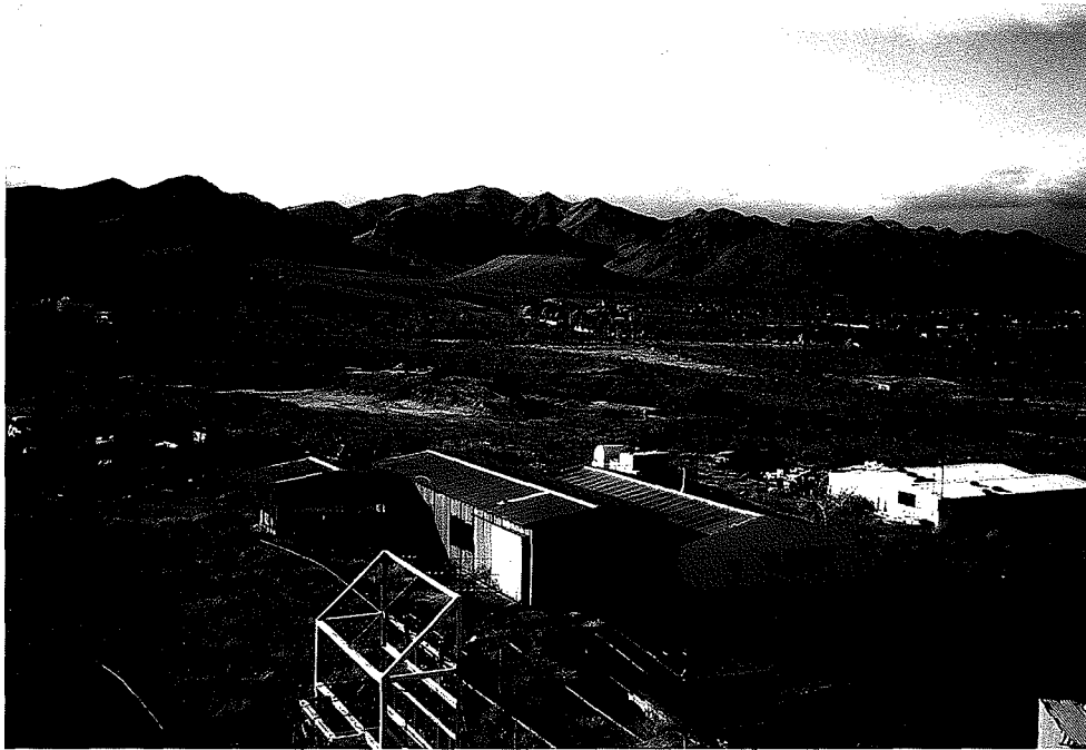
The mining and milling plant of radioactive mineral at Villa Aldama and the tailings impoundment (Spain).
