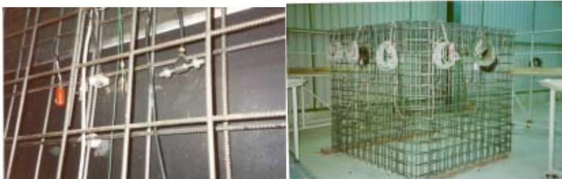
**Figure 3:** Preparation of the embedded sensors in El Cabril
