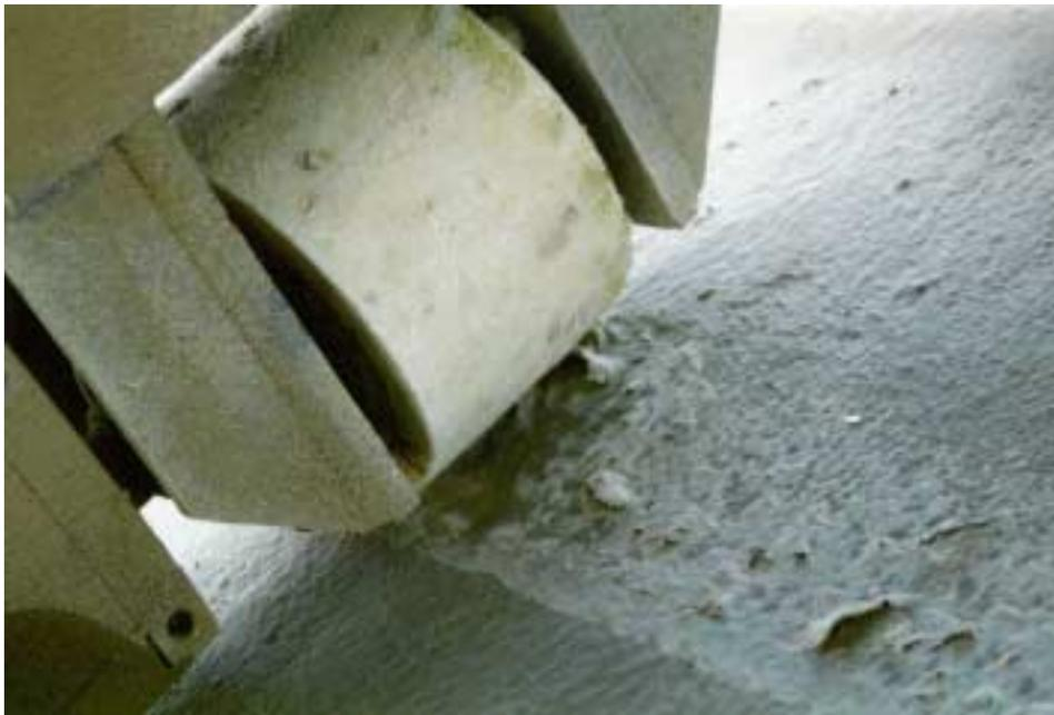
Picture 5: Damages on the repair system caused by high load on scaffolding wheels
