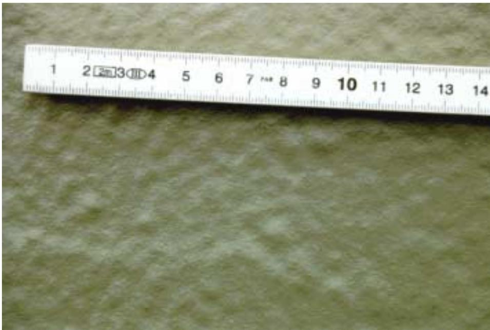
Picture 8: Perfect surface of the crack overbridging surface protection system
