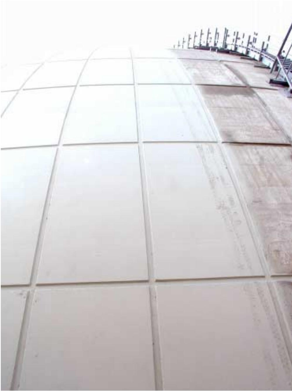
Picture 4: Dome with fluting structures
