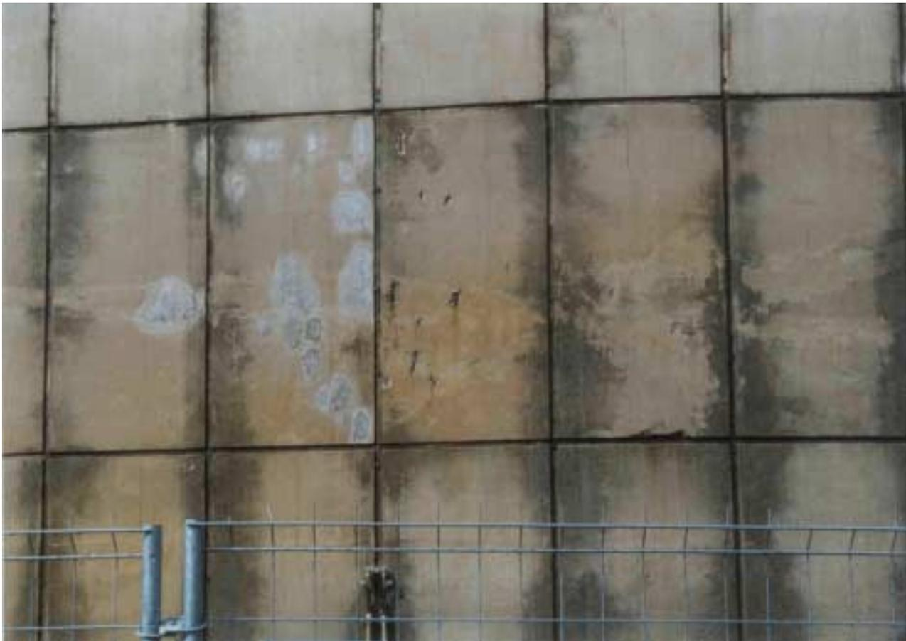
Picture 2: Concrete surface of a safety compartment with damages and deteriorations
