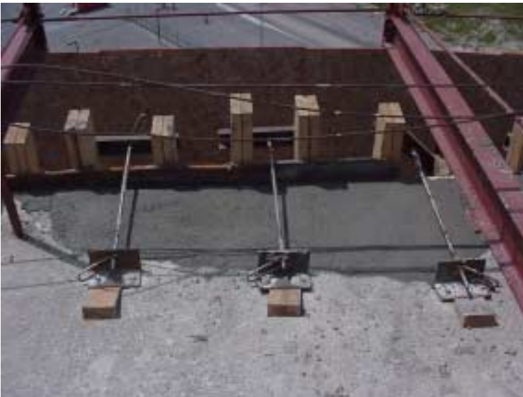
Figure 10: Deep Repair – Completed
