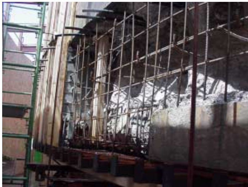
Figure 7: Installation of Skin Reinforcement
