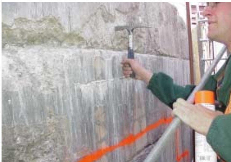
Figure 5: Sounding the Concrete Surface
