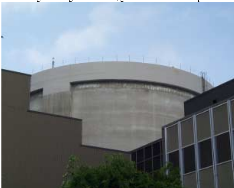
Figure 13: Completed Repair South-West View
