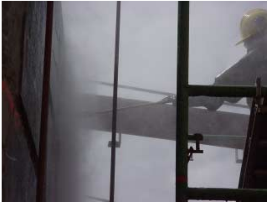
Figure 8: Surface Preparation –Hydro-Jetting
