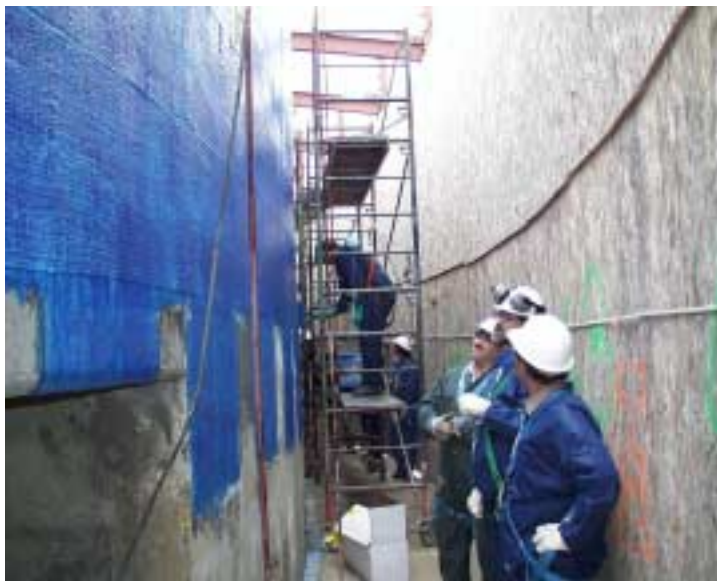
Figure 11: GFRP Installation
