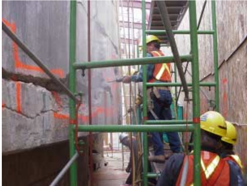
Figure 6: Concrete Demolition
