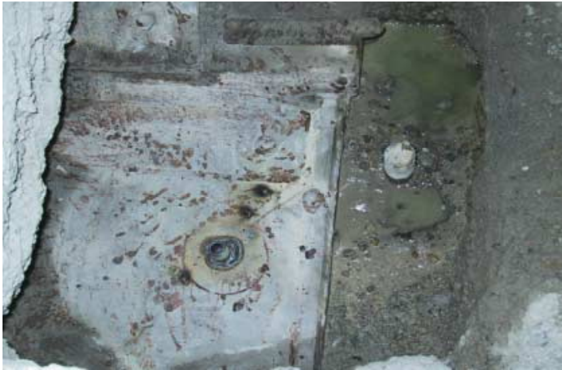
Injektion point No 1./19 with injection cap
