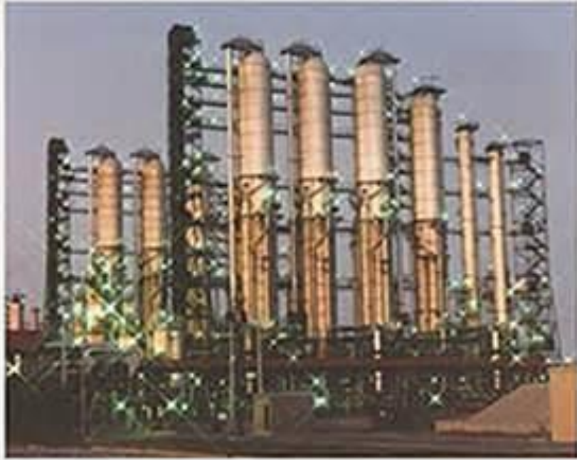
Bruce Heavy Water Plant
