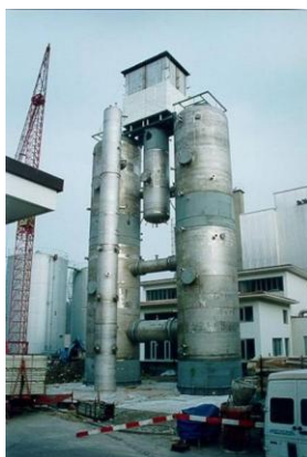
PANDA vessel assembly (construction phase, 1993)
