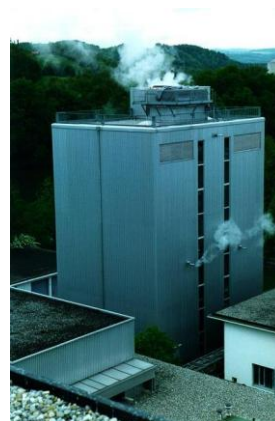
PANDA building (whilst performing a test)
