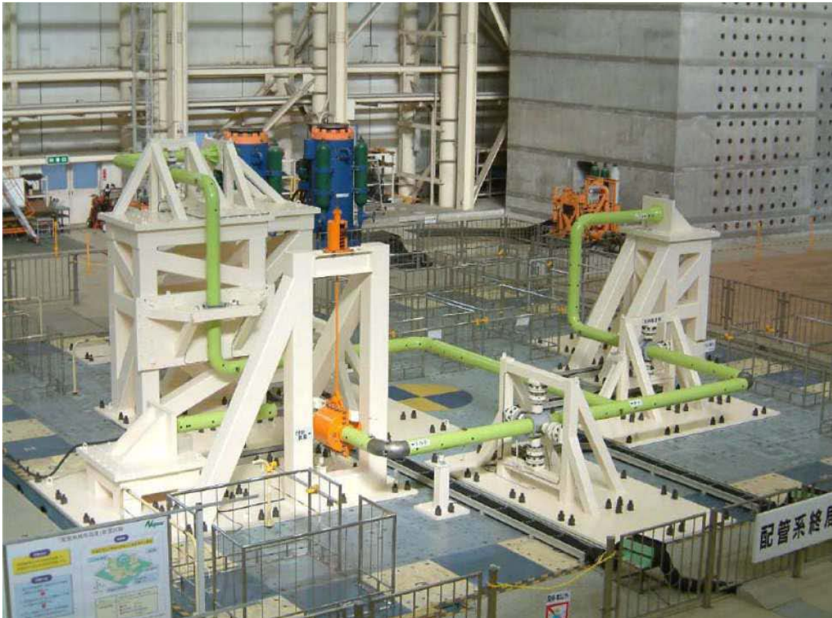
Figure 5: The NUPEC piping system on the Tadotsu shaking table
