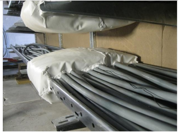
Figure 26: Wrapping of the fire barriers by a cloth
